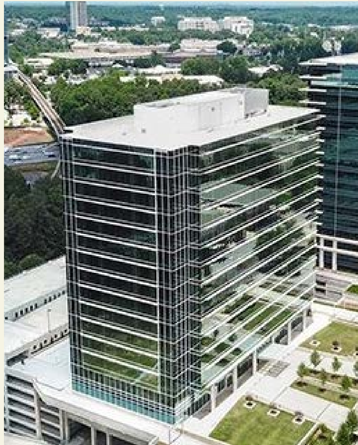
Developed 4004 Perimeter Summit Central Perimeter - Atlanta 350,000 SF
